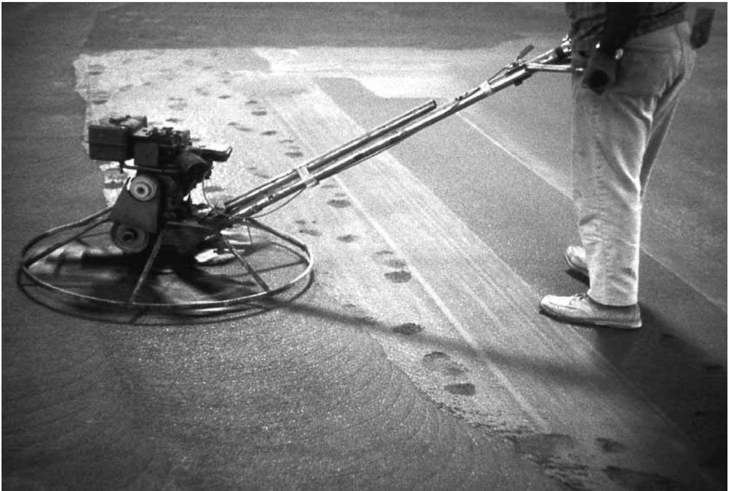
Power floating a screed.
